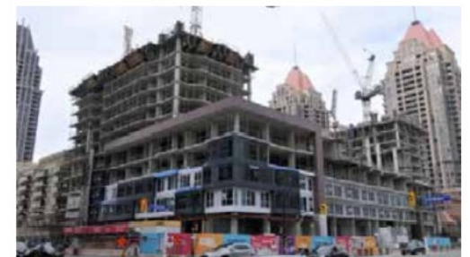
Mixed-use high density construction near HMC
